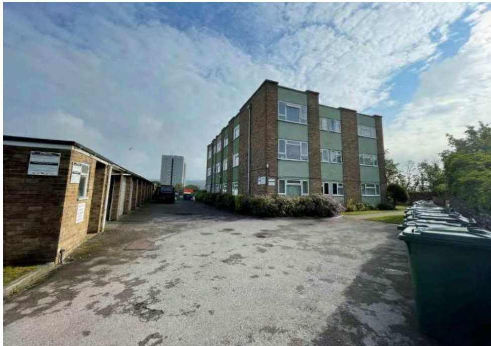
Photo taken from the top of the entrance road looking North
